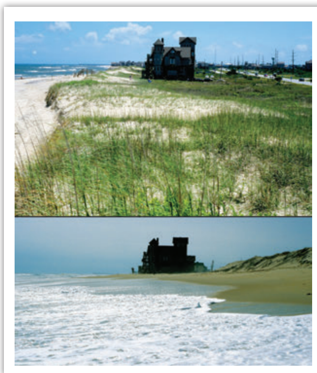
Continuing Erosion in Rodanthe, North Carolina ©Gary Braasch 2014
